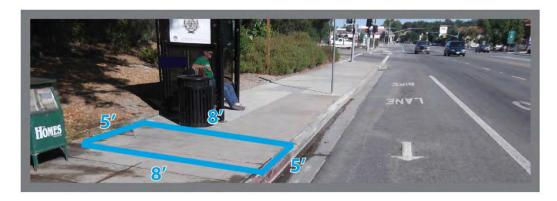
The graphic above shows the minimum dimensions of the width and length for a mobility device landing pad on existing bus stop.
